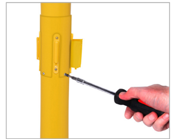
Step 1: Remove post retaining screws
